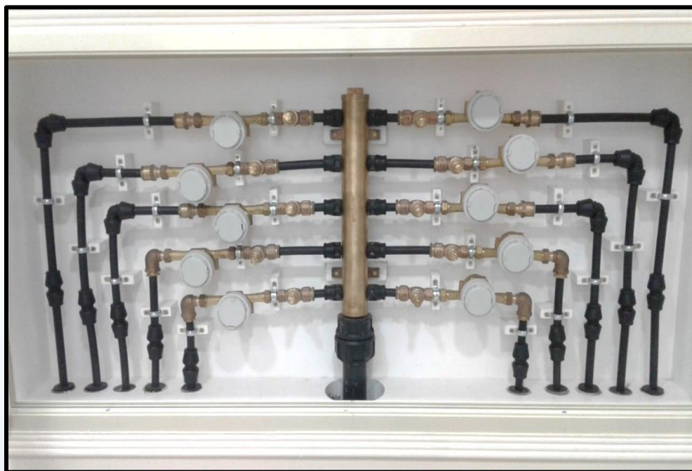
Figure 7. (50mm) manifold
