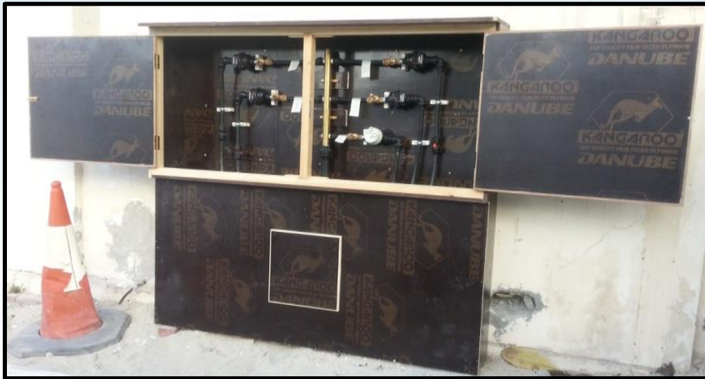
Figure 8. (25mm) manifold
